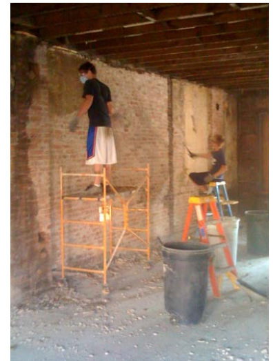
Right: Participants repair masonry preparation for complete rehabilitation of this historic unit across from Prescott School in Dubuque.
